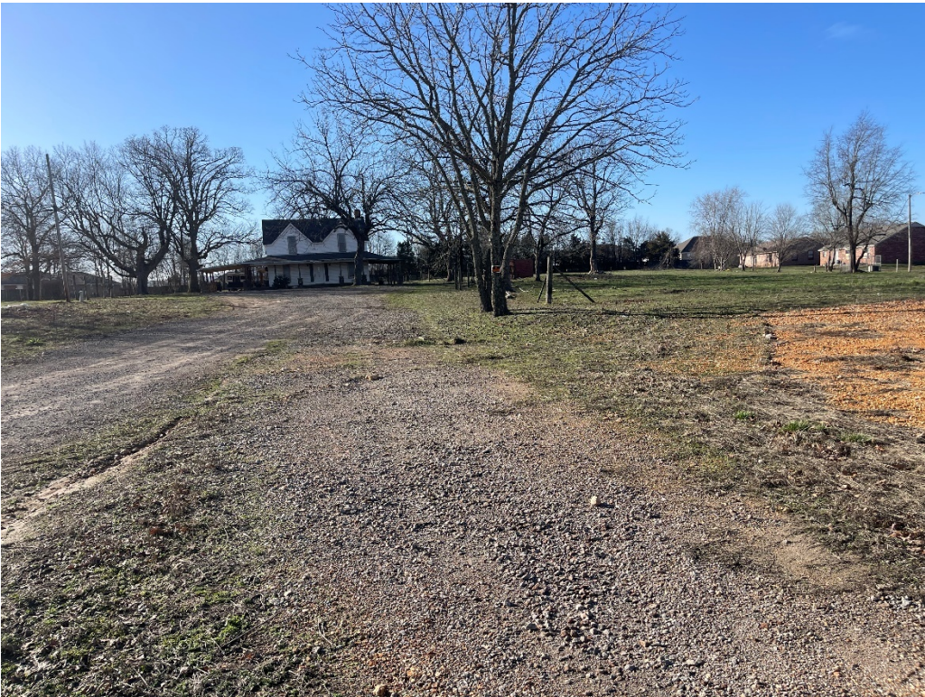
Figure 2: View looking south, towards the existing building
