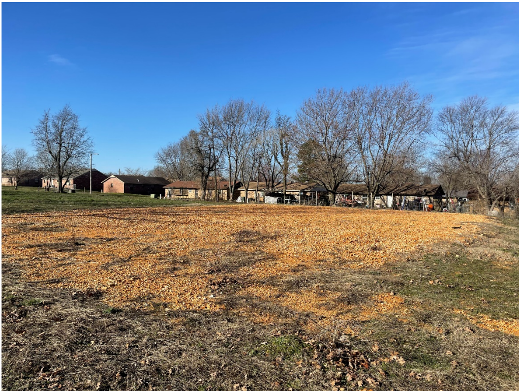
Figure 5: Chert gravel exposed within northern portion of planned construction area
