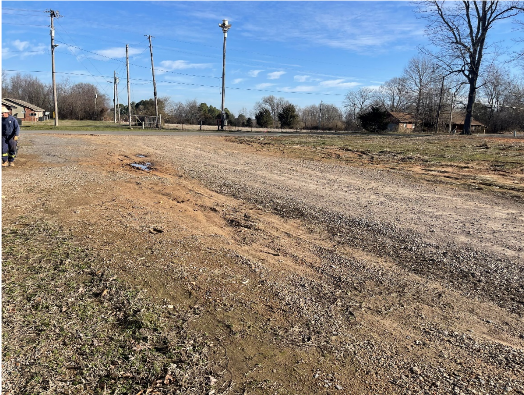
Figure 4: Ponding water within the existing gravel drive area
