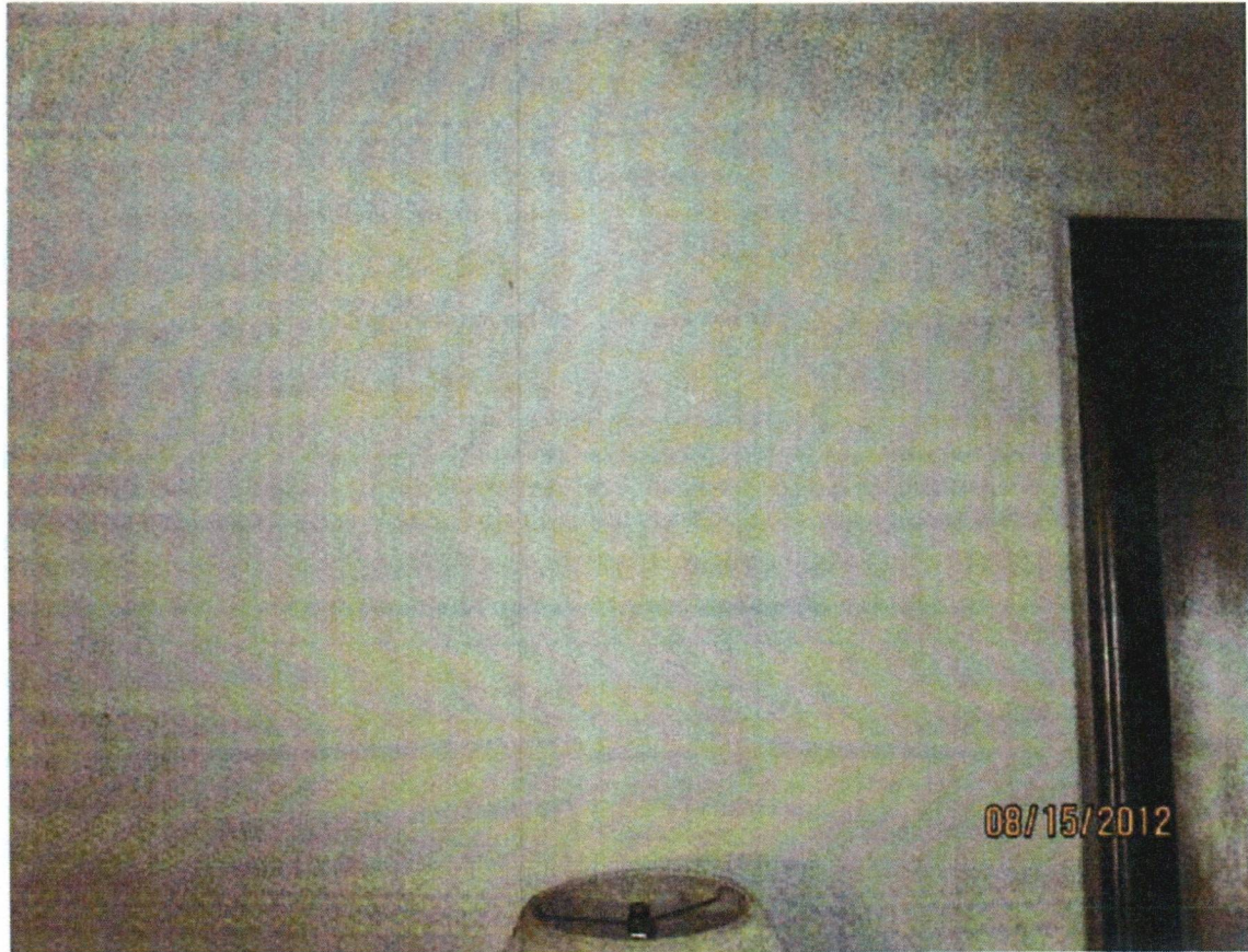
Living Room Joint Compound (2%) Chrysotile Asbestos
