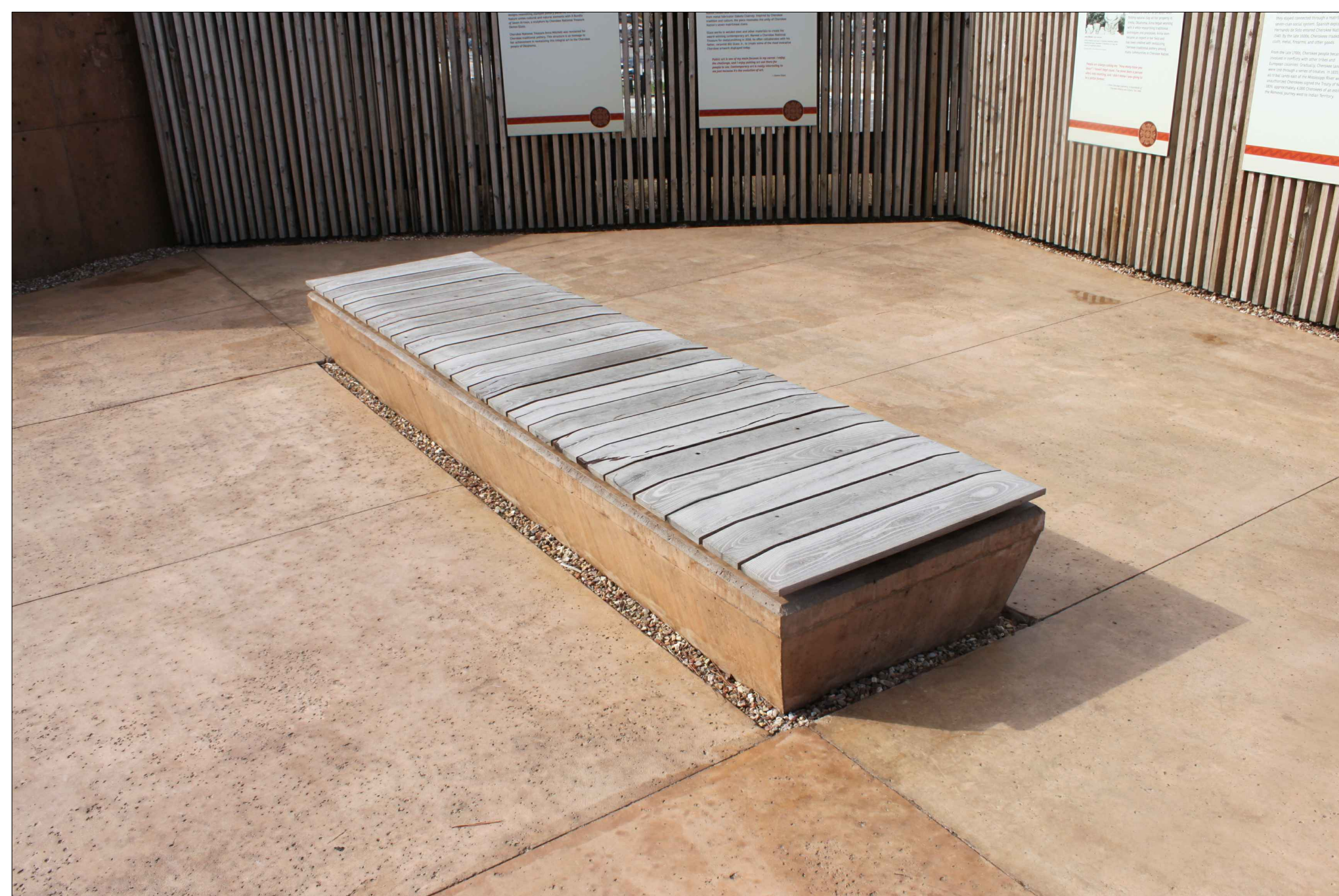
EXISTING CONCRETE BENCH - FOR REMOVAL
