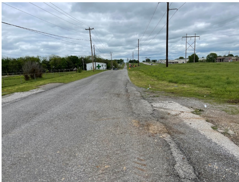
Figure 3: East end of the existing roadway, facing west
