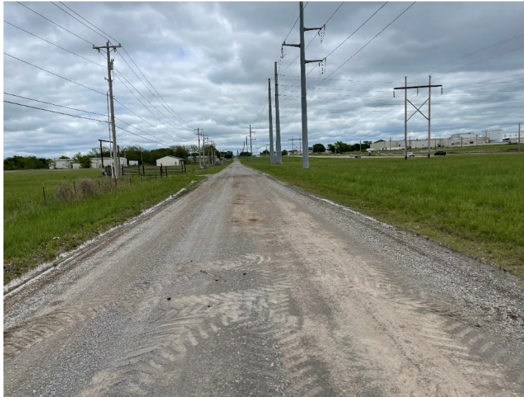
Figure 4: West section of the existing roadway, facing east
