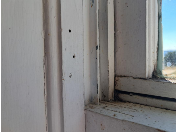
Existing Historic Window Stop Molding
