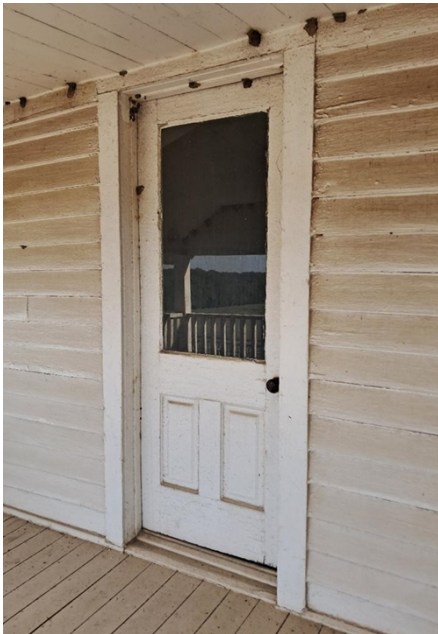
Existing Sleeping Porch Historic Door
